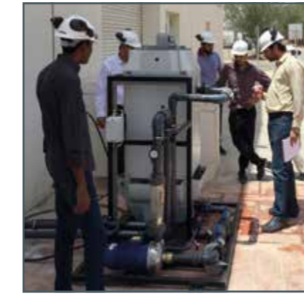
Inspection of the plant on site
