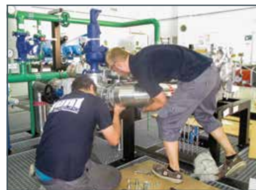
Assembly of the centrifugal pump on site
